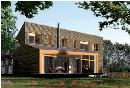
Passive energy home of M. Damico in Le Mesnil-St-Denis.
